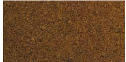
40T1C00 Finished tiles
